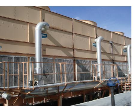
Cooling tower coatings need to withstand extreme environments, including immersion in water, exposure to corrosive chemicals and temperature extremes.
