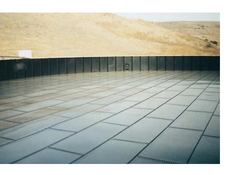
IT Corporation in Benecia, California learned that the leachate being stored in its two 150 foot diameter tanks had damaged the tanks' epoxy liners and was leaking.
