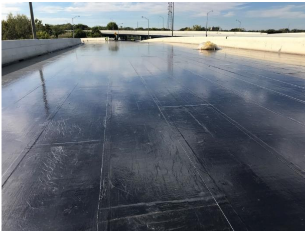
Fig. 1 Completed Membrane Installation
