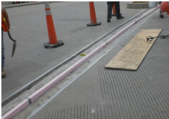
Fig. 2: Insulation Board used in joint opening
