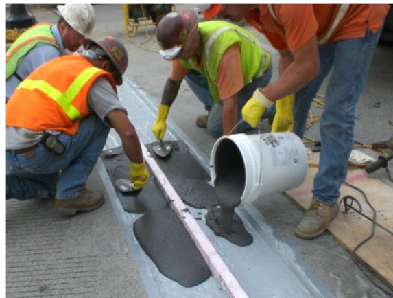
Fig 3.1 ECCrete 57N Installation
