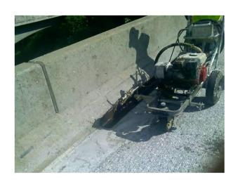
This overbanding of all surface joints (longitudinal and transverse) should be done at the completion of paving, so long as it will not result in any safety related issues.
